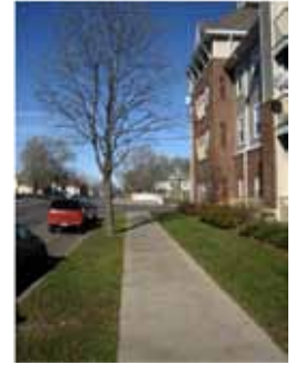
A new sidewalk in front of the 2909 Apartments.
