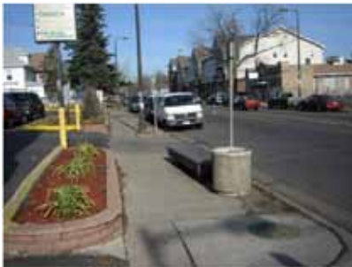
Existing landscaping and pedestrian facilities outside Super Mercado La Mexican.
