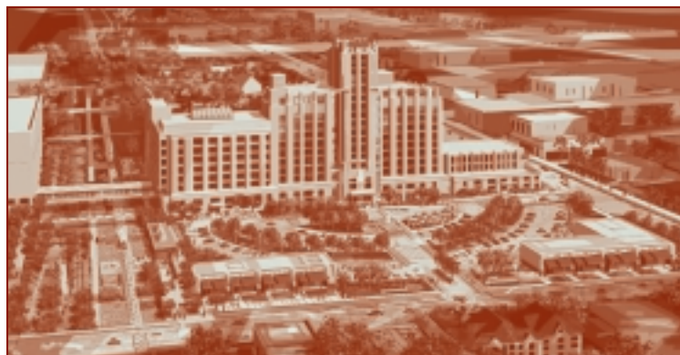
The former Sears site in South Minneapolis, seen redeveloped as the Midtown Exchange. Courtesy Ryan Companies
